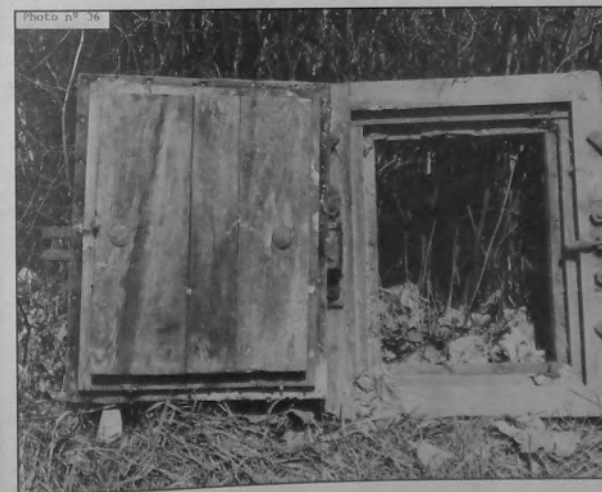
Photo 36: PMO II-5-64/2 with its «door» open. In order to make it gas-tight, two bands of felt were nailed to the door and the frame (strips of felt can still be seen on the frame).
