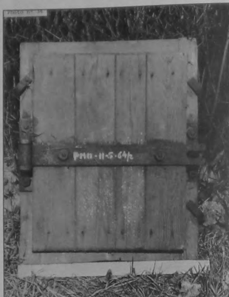
Photo 34: Outside of PMO II-5-64/2, of the second pattern, door 40 by 50 cm, in excellent condition.
