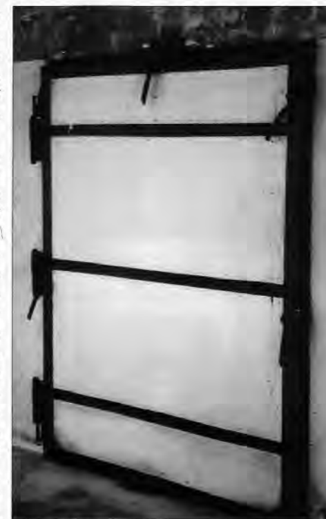
Figure 71: Gastight, escape-proof steel-frame door to one of the Degesch circulation delousing chambers at the Buchenwald Camp. (© C. Mattogno)
